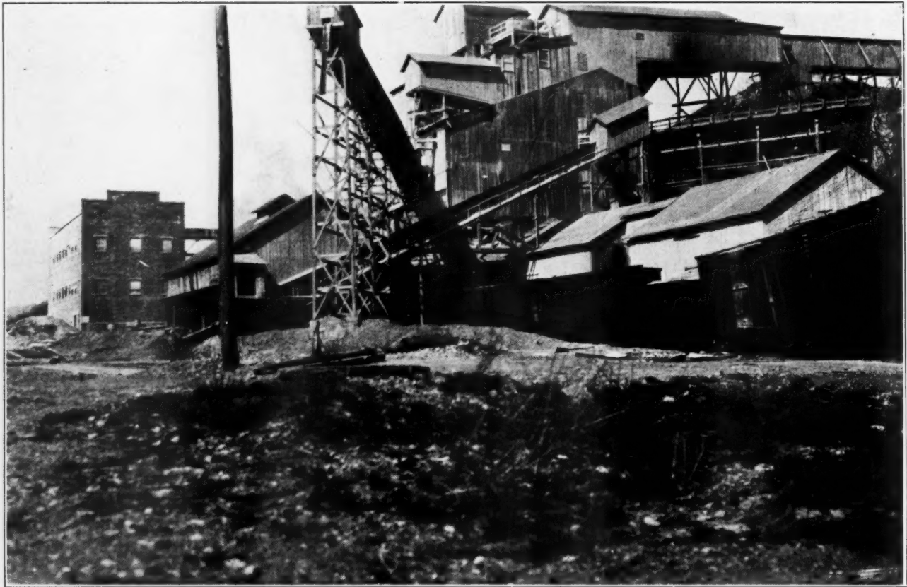
The Secondary Crushing and Screening Plant. The Overhead Discharge Conveyor in Foreground is for Chips. The Hydrate Building is Shown in the Left Background.
